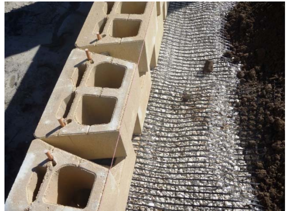
Figure 1. Miragrid® 5XT in SRW.
