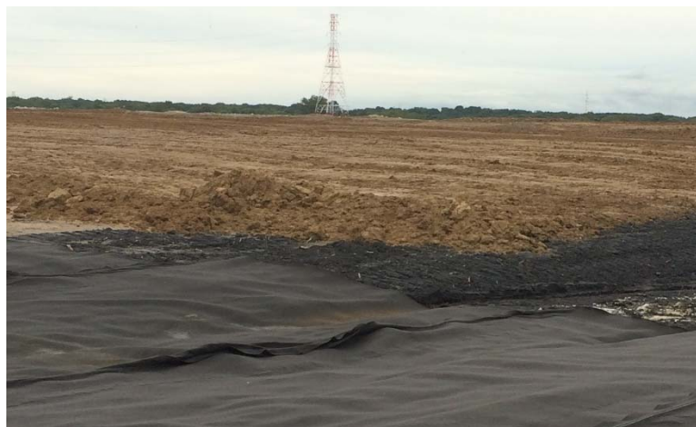
Figure 10. Construction resumes following pore water dissipation.
