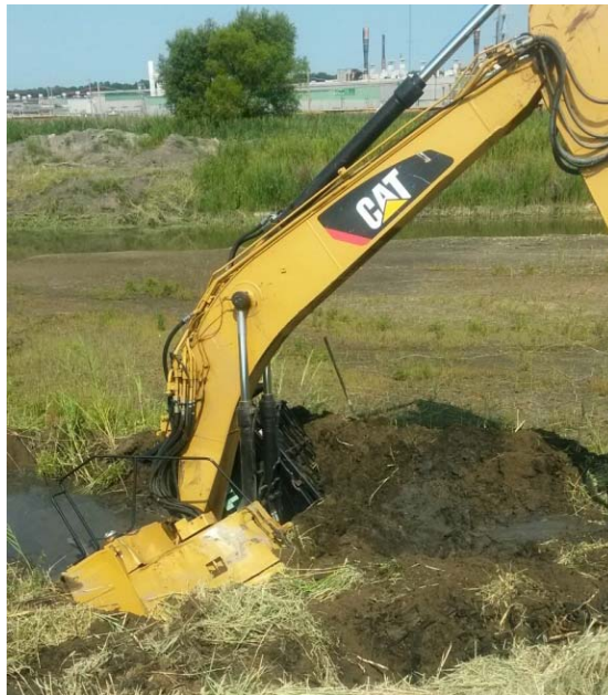
Figure 1. Soft, saturated CCR subgrade soil below surface crust.
