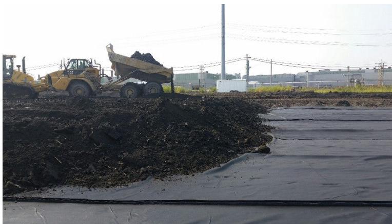
Figure 8. Fly ash fill placed on sewn, geotextile panel.
