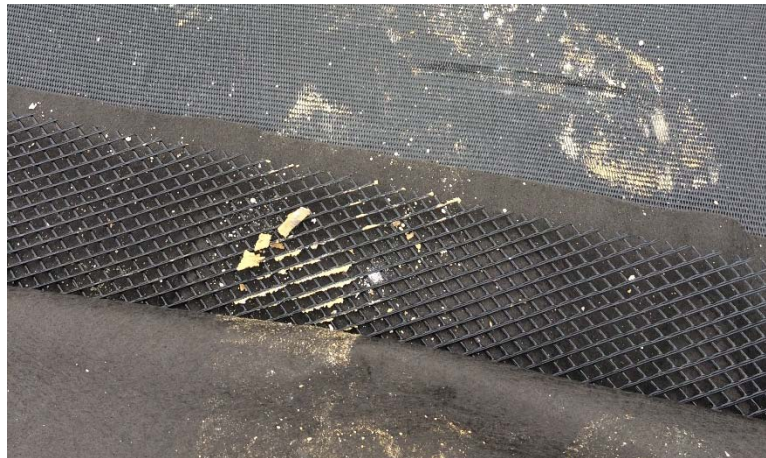
Figure 9. Geocomposite drainage layer laid directly on top of the geotextile.
