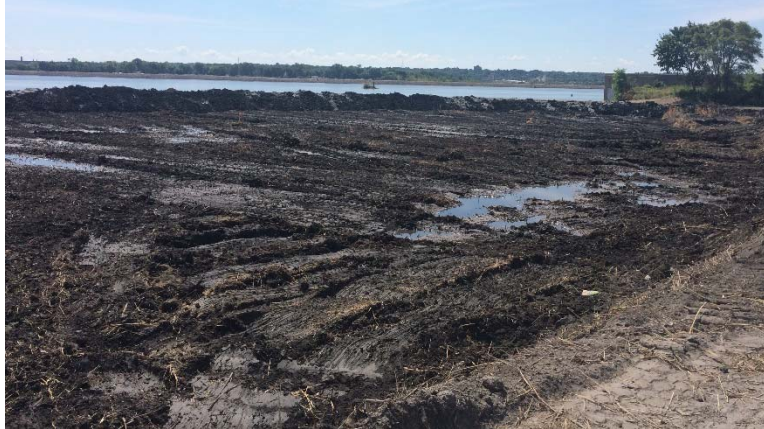
Figure 2. Clearing operations completed.
