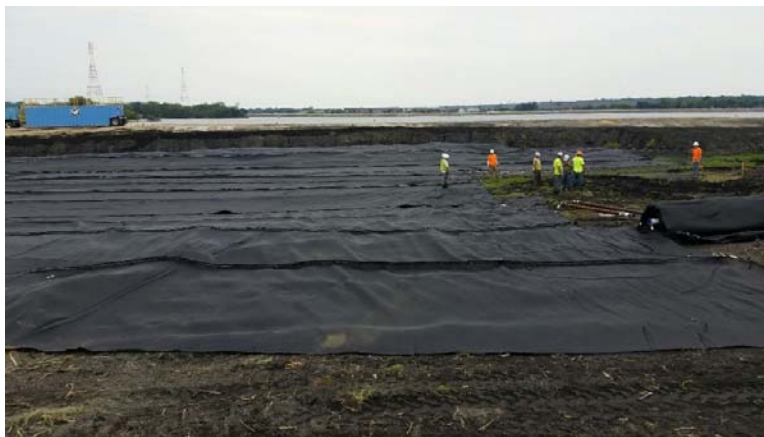
Figure 7. Sewn geotextile panel deployment.
