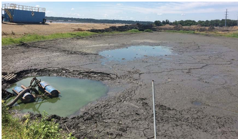
Figure 3. Surface water removal.
