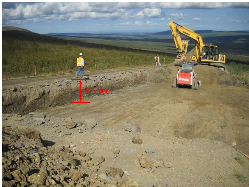
Figure 1.1 Excavation of East Lane (Looking North)
