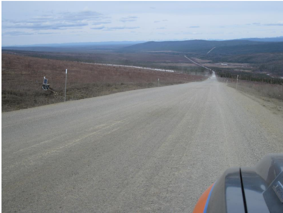
(b) Road conditions On May 24, 2011 (After Treatment)
