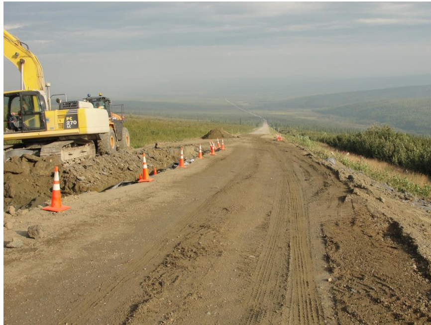
Figure 3.5 East Lane of Road after Construction
