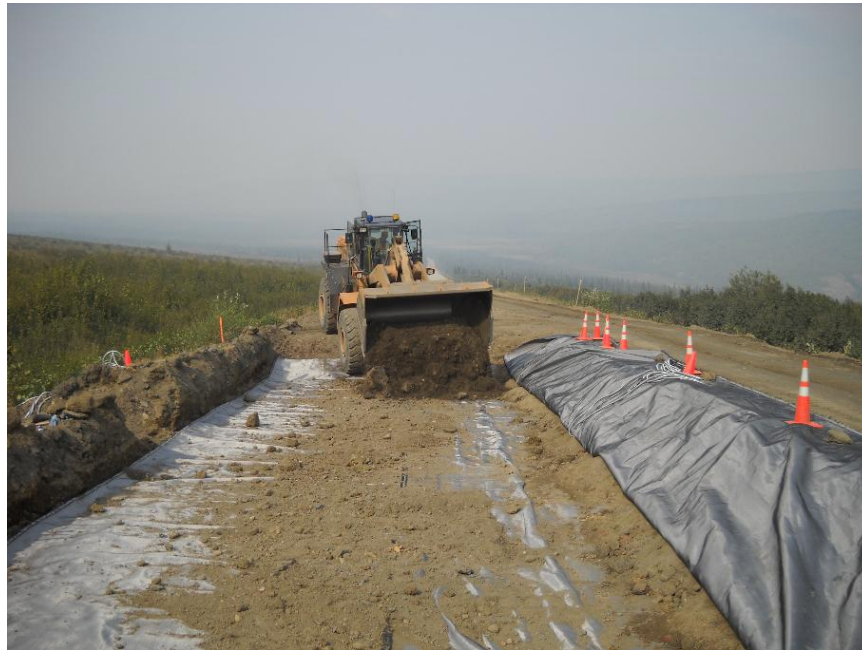
Figure 3.7 First Layer of Wicking Fabric on West Side of Road
