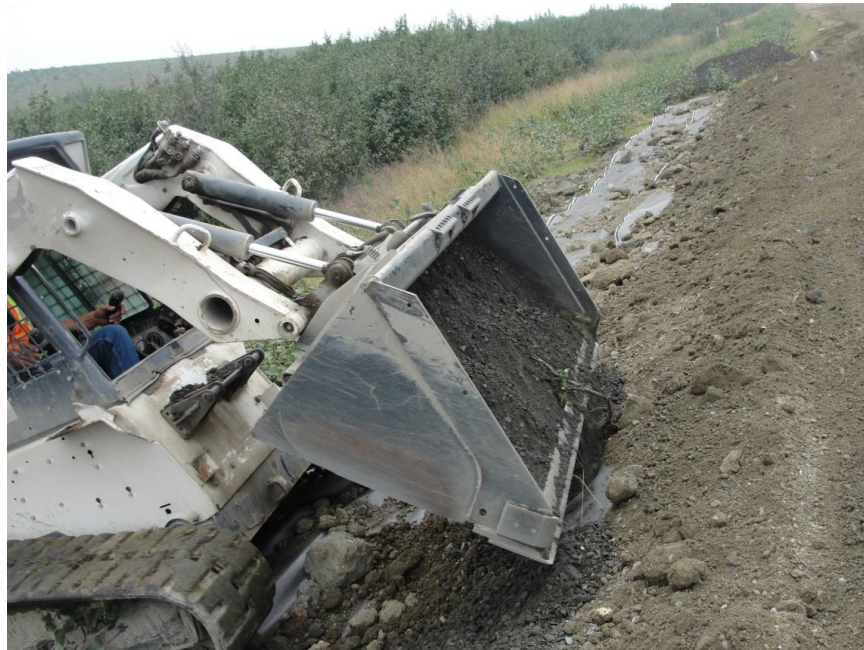
Figure 3.8 Covering Wicking Fabric with Crushed Rock at the East Shoulder
