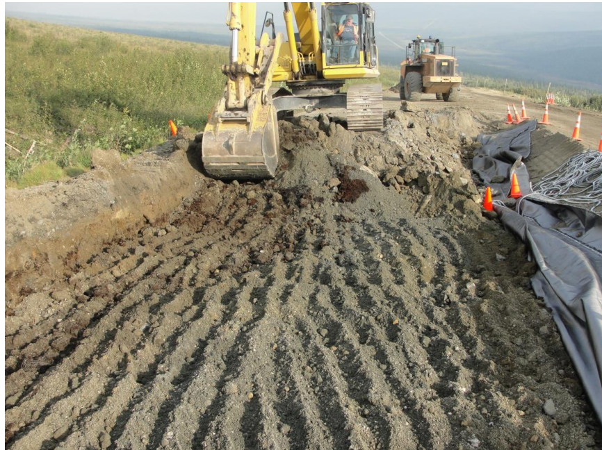
Figure 3.6 Excavation of West Lane of Road
