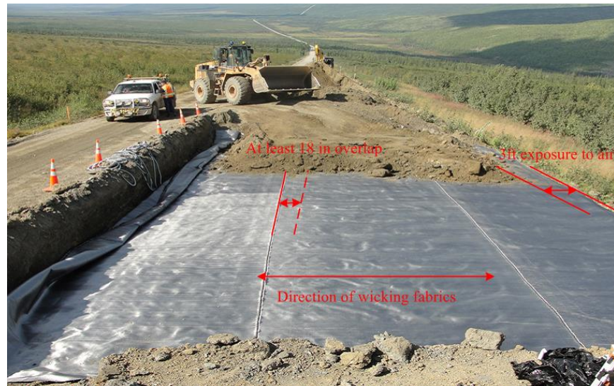
Figure 3.4 Bottom Layer of Wicking Fabric after Placement
