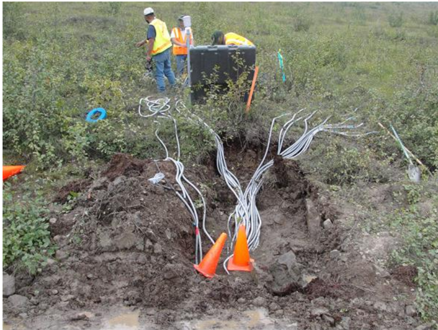
Figure 3.9 Construction of Data Collection Station
