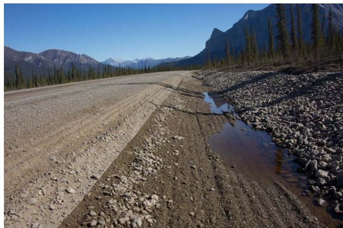
Figure 10. Performance of the wicking fabric geotextile in the Dalton Highway project
