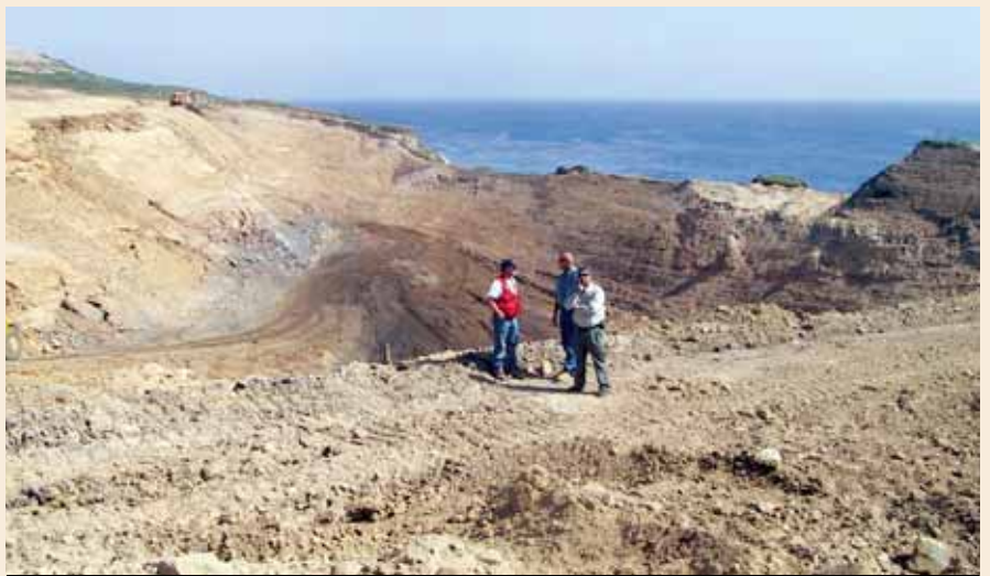
Photo 2. Initial stabilization work involved extensive earthworks.
