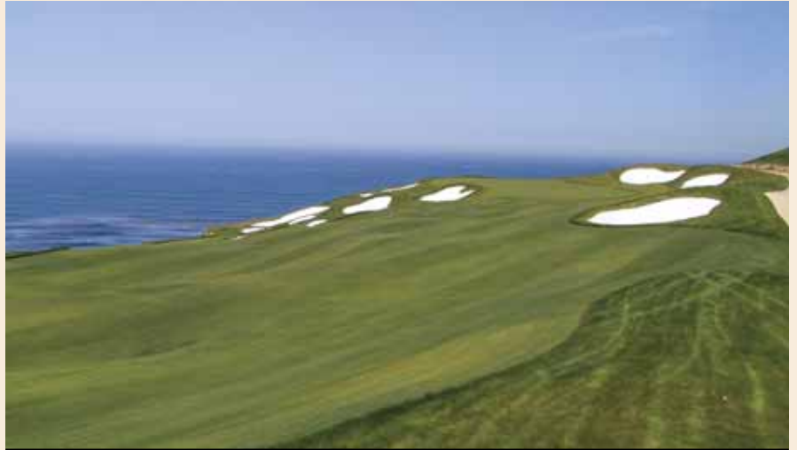
Photo 1. A landslide took out most of the 18th hole. The rebuild created a signature hole and a signature geotechnical design.
