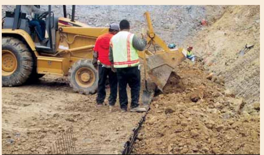
Photo 4. Constructing the geosynthetic-reinforced MSE wall buttress.
