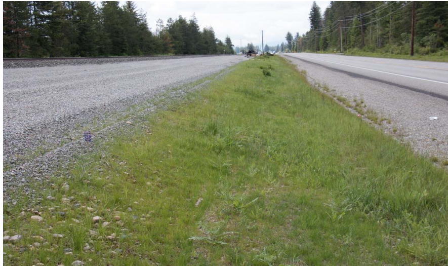
Image 11 - Native Plants Establishing the First Season after Installation
