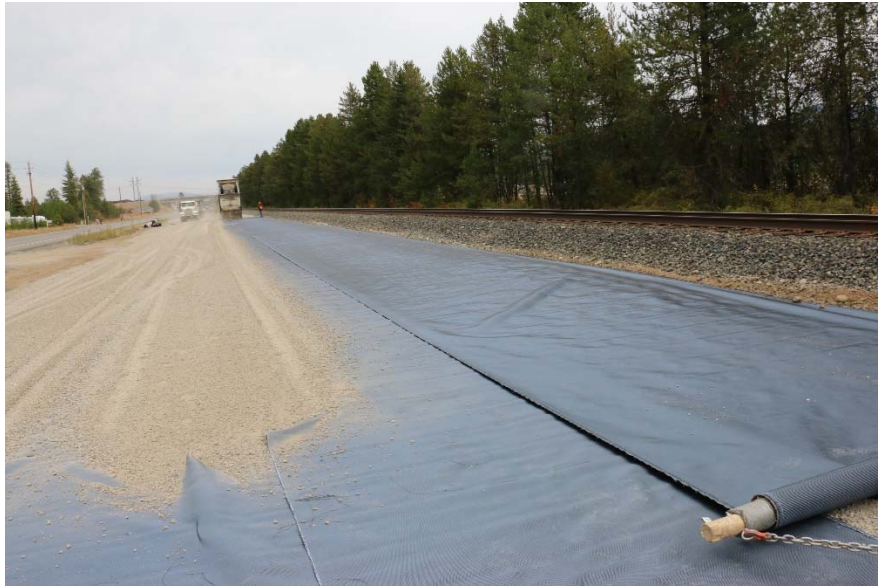
Image 16 - Forklift Pulling the Material Taught as Truck Begins its End Dump.
